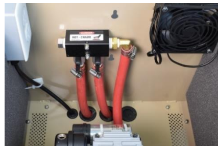
Manifold after connections
