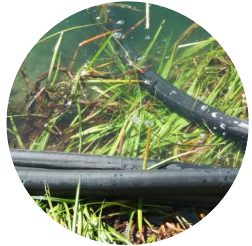
Torpedo hose in a pond connecting Bubble Tubing® lines and the compressor.
