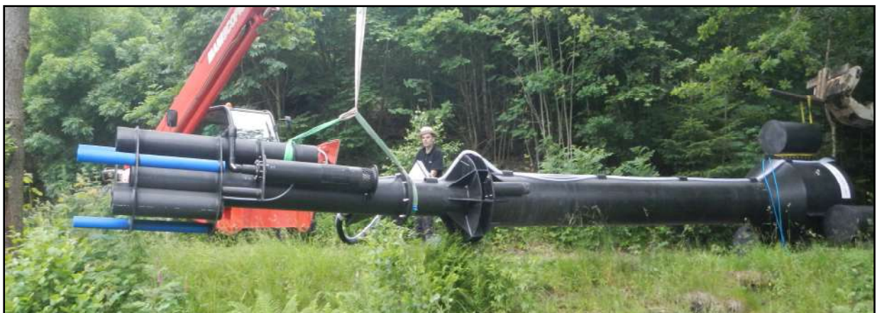
Fig. 7: Installation of the first plant
