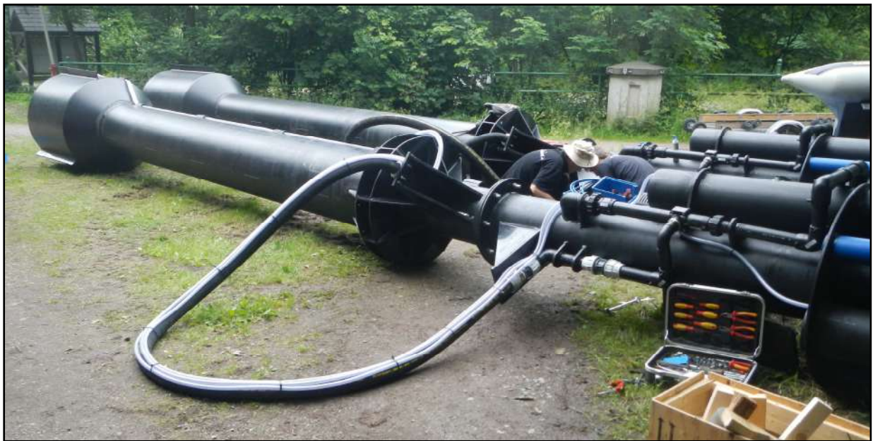
Fig. 6: Final on-site mounting: telescopic element
