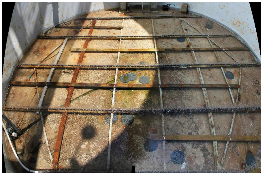
Figure 2-2 - Photo of typical Bubble Tubing™ Arrangement
